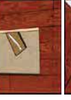
Picture 7: Preparation of layers is done by spreading glue on a trim laminated foil, or on a piece of veneer, first spreading the glue on veneer below the neighbouring boards, and after that spreading glue on a part of veneer which should fix the new board.
