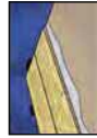
Picture 7: Angle the next board into place along the short end. Then push the board until the long side is in place in the groove. Do not press the board down into the adhesive. Continue in the same way with the next board until the whole row is in place. Lay the board in place in the groove without pressing it down.
