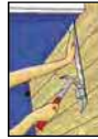
Picture 12: Our adhesive, lay the last row of boards and tap them into place using the pull bar.
