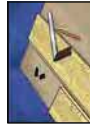
Picture 4: Cut the board to the right length with a handsaw (from the top of the board) or a circular saw (from the underside).
