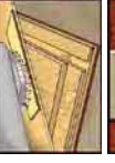
Picture 6: The new board that will be installed, must be prepared first. After you checked the board size, saw off the underside of the short ends and long side, but be careful not to damage top surface and not to remove board tongue.
