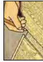
Picture 3: At the end of the row, turn the last board so that it ties tongue to tongue. Push the short end tightly against the wall. With a pen, mark where to cut 8-10 mm from the end of the previous board, to make it easier to get the board into place.
